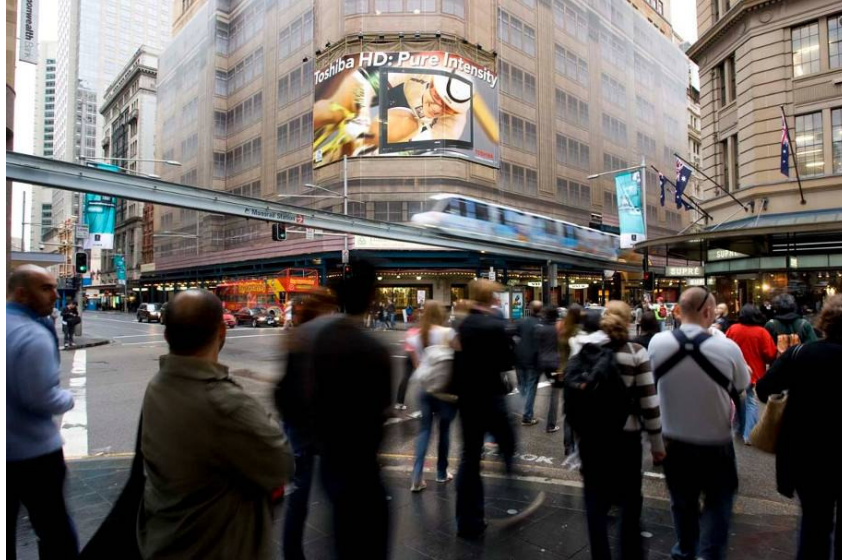
Figure 1: Building wrap corner George and Market Streets, Sydney
